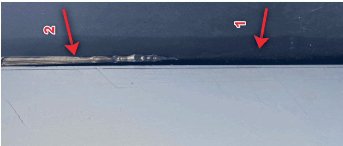
Figure 40 Correct application of 418 urethane at Arrow 2
